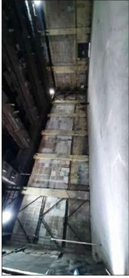
VEGETATION CLEANING, REMOVING WALL CLADDING, OLD ACOUSTIC PANEL, CORROSION ON STEEL MEMBERS
